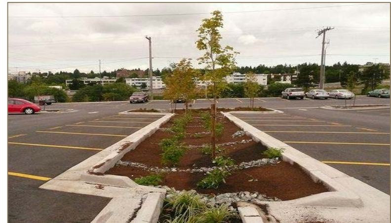
NE Siskiyou Green Street Project; Pervious Pavement Projects City of Portland
