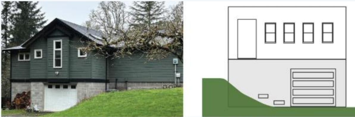
Figure 8. A Building Elevated on an Enclosure used for Parking
