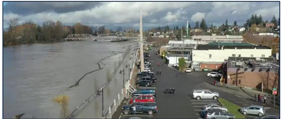
Figure 1: Skagit River flood wall in Mt. Vernon WA, November 16 th , 2021.
