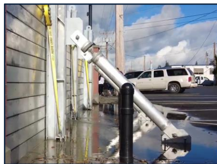
Figure 2: Flood wall braces in Mt. Vernon, WA.
