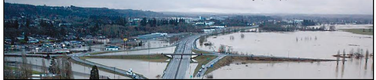
Flooding across U.S. Interstate 5 near Centralia, Washington, January 8, 2009.
