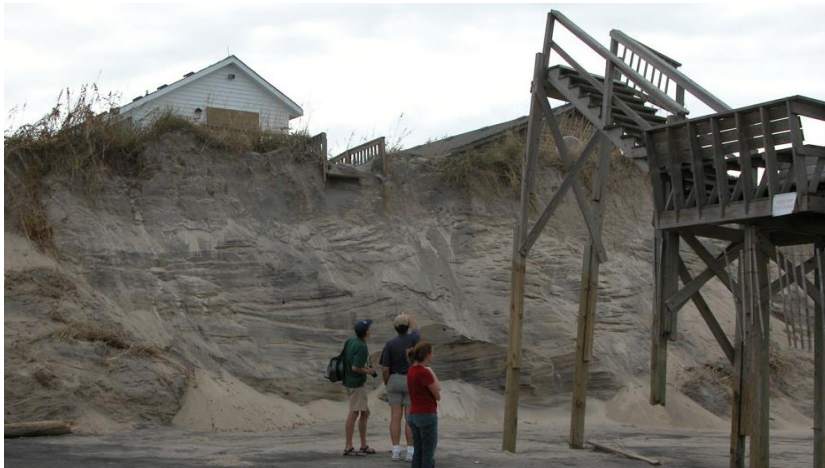
High storm surge and wave runup during Hurricane Isabel caused widespread dune erosion in Nags Head, NC.
